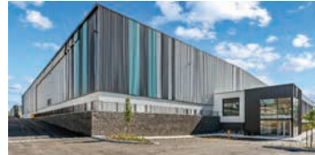
100 Metroplex Place, Wacol, QLD Completed June 2022 Fair Value 1 $45.4m | GQLT (GPT 50.1%)
