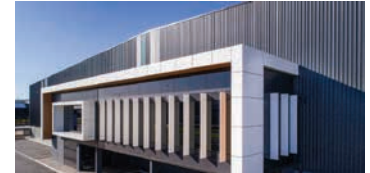
143 Foundation Road, Truganina, VIC Completed July 2022 Fair Value $23.4m | GPT 100%
