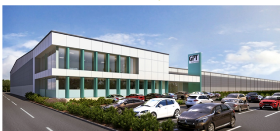
Eastern Creek Drive, Eastern Creek
